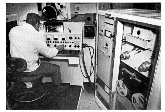
ELECTRON BEAM welder becomes a versatile tool when coupled to numerical tape control unit (right). Jim Taylor (4221) operates the newly-operational equipment which was designed specially for Sandia. The operator manually programs a weld path for each part to be joined and the numerical tape control then drives the welder when the tape is played
